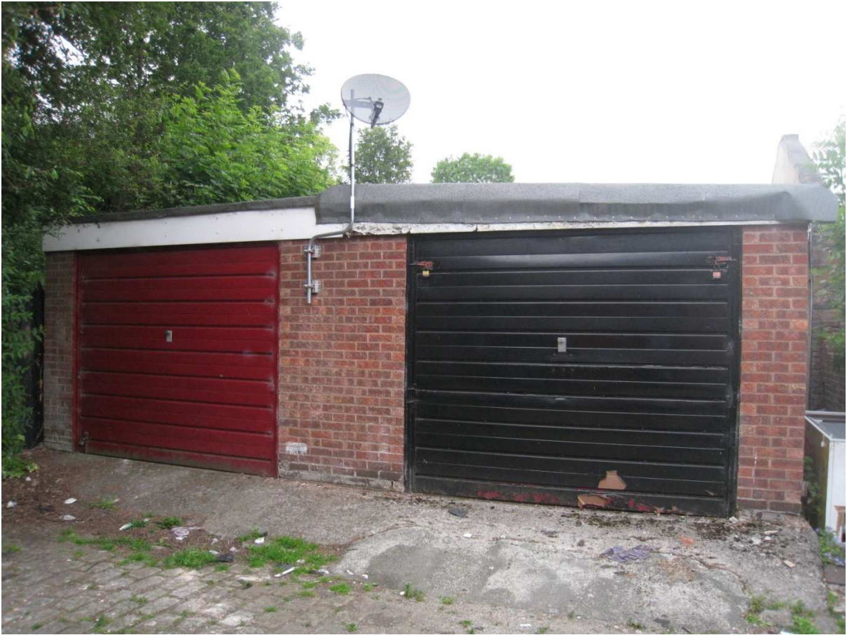
Satellite dish on roof of garage
